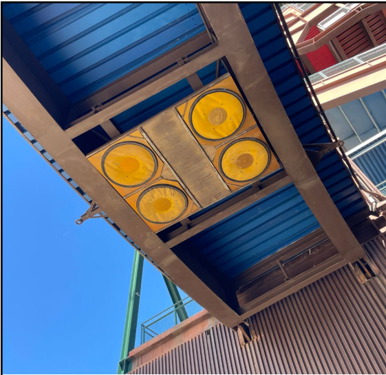
Figure 15: Air movement system ball bearings visible on underside of pedestrian bridges.
