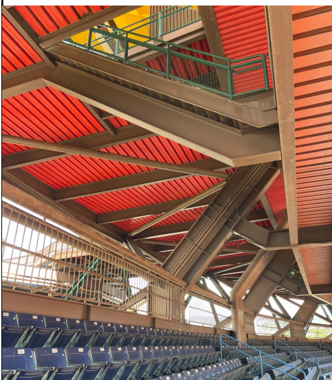
Figure 5: Corten steel structure supporting the upper tiers of the stadium. Replacement railings visible in upper tier.
