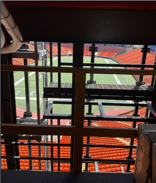
Figure 36: Scoreboard support structure.
