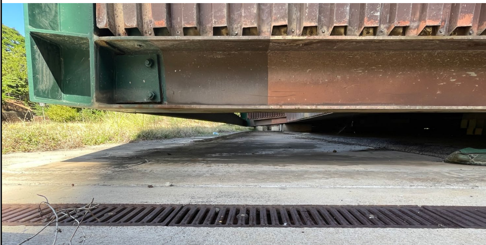
Figure 16: Base of moveable stadium section hovers above cement movement pad.
