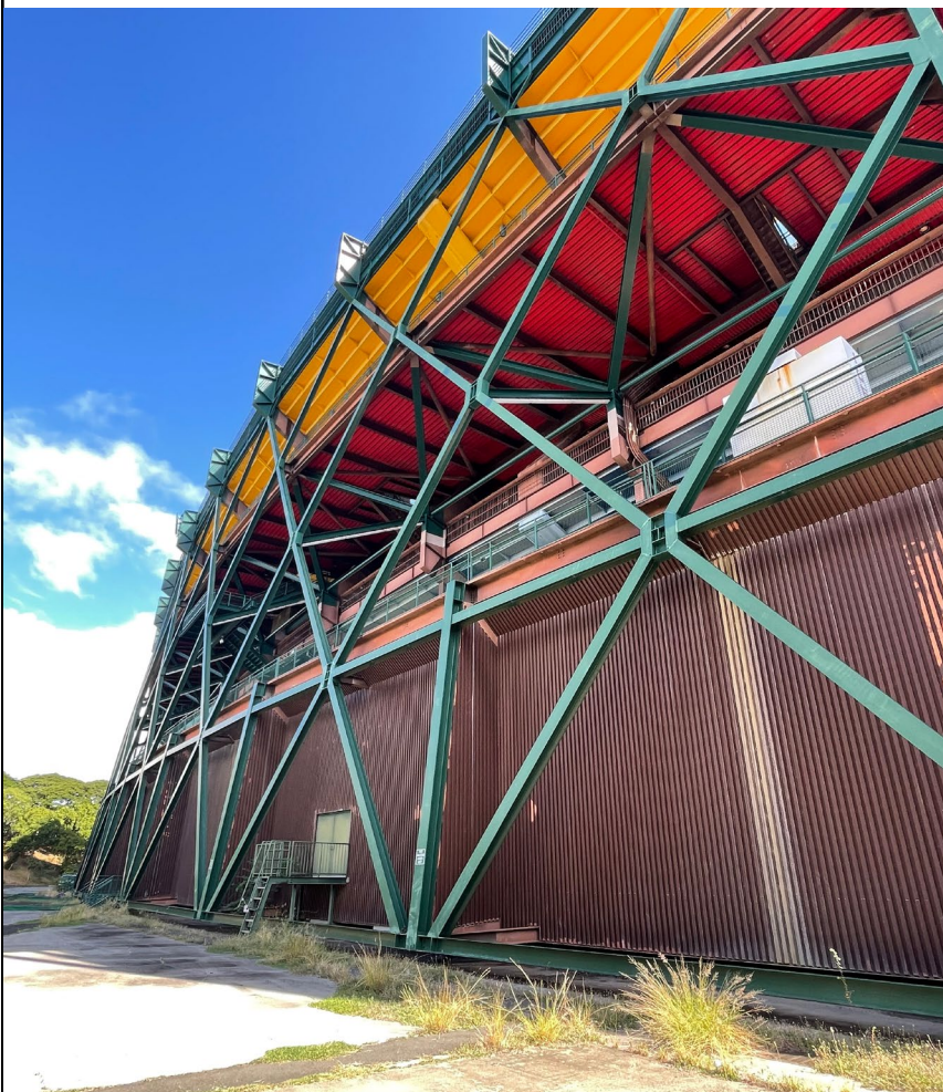
Figure 2: Exterior of stadium at southwestern corner. Corten steel structure is visible as well as ribbed steel walls around base.
