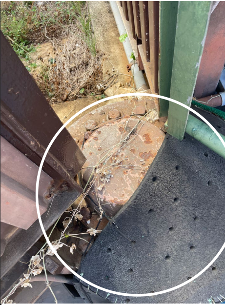
Figure 18: Massive hinge where moveable and stationary stadium sections meet.
