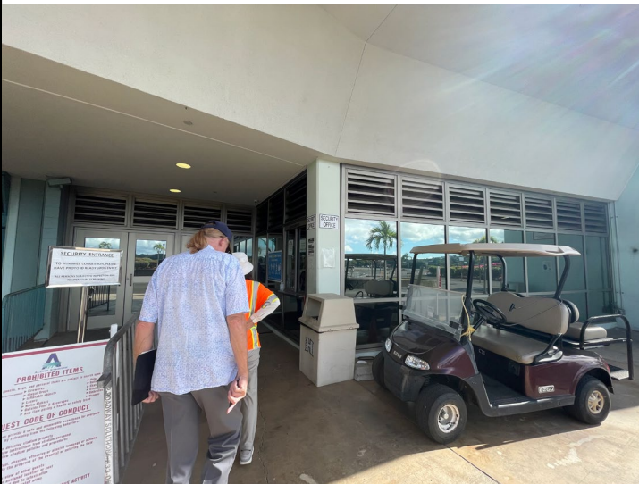
Figure 28: Infill windows and doors in eastern bay of box office & stadium main entrance.
