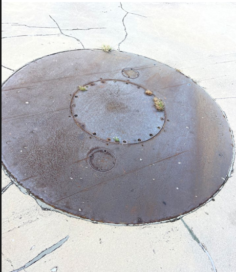
Figure 19: Piston cover for pedestrian bridges.
