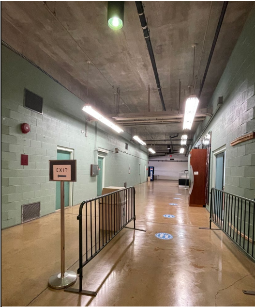
Figure 30: Interior hallway behind box office showing concrete block walls, finished concrete floors, and exposed utilities on ceiling.
