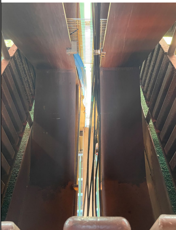
Figure 17: Meeting point of two moveable stadium sections showing corten steel structure.
