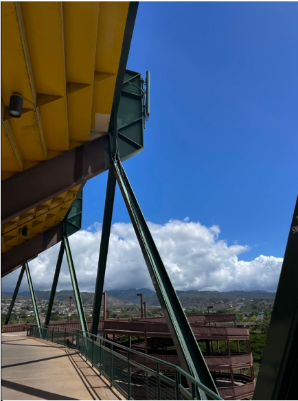
Figure 6: Pedestrian exterior walkway along upper tier showing replacement railing and corten steel structure.
