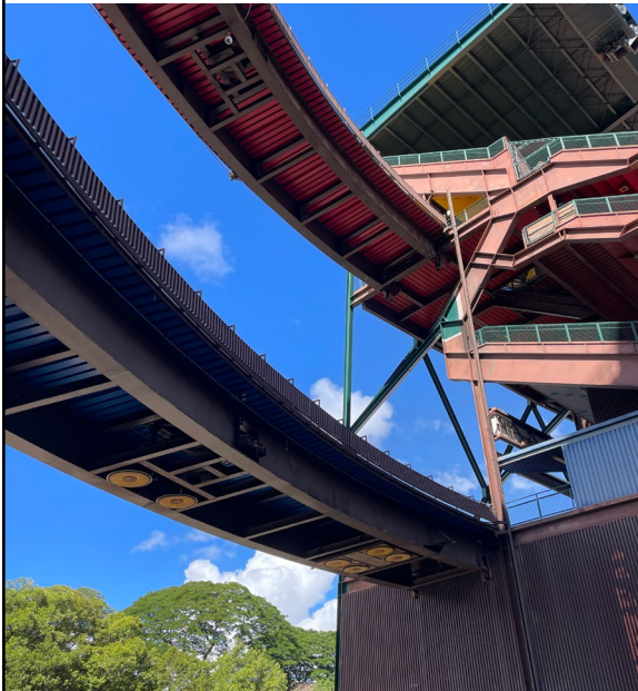
Figure 13: Moveable pedestrian walkways at southwest corner of stadium. Moveable walkways are found at four corners of the stadium.
