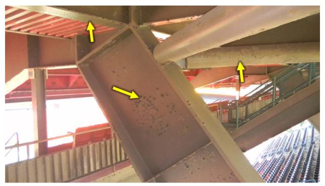
Figure 9. Example of structural steel member classified as Condition State 2
