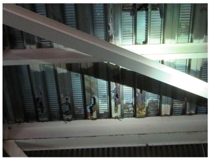
Figure 14. Example of lightweight floor slab decking classified as Condition State 4.
